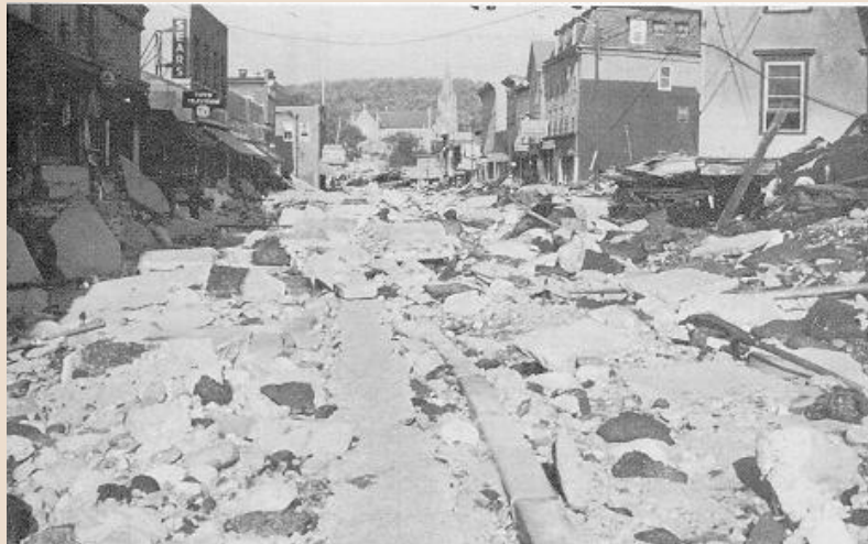
Winsted, CT in 1955 after hurricanes Connie and Diane caused a dam to fail. Waterlines on the 3rd floor of old mill buildings could still be seen many years later.
